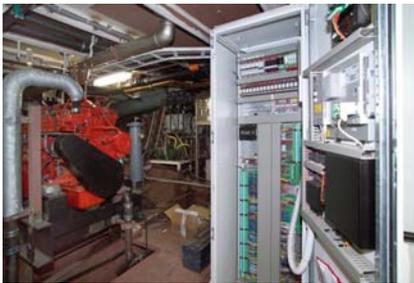
Four S-MAX controllers are being used in the 'Boreas'. Using PROFINET these exchange data transparently with other equipment such as the motor management and fire alarm systems. PROFINET is certified for shipping and it handles the data transported between the PLC and the I/O modules and the normal
